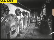
In 1893 the Campolmi clipping factory had two Cornwall model boilers formed by a large water tank heated by an internal fireplace. In 1925, the system - currently visible in the Museum - , built in refractory material, was purchased,. The plant, modified several times, was intended to produce energy to operate the textile machinery.
